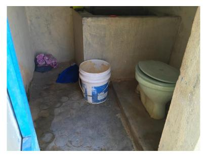
Picture 9 Some persons with disabilities have retrofitted western water closets.A water storage tank is constructed behind the water closet.
